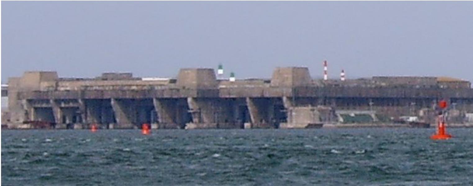
Germans built these U-Boat pens using forced French labor at Lorient on the north coast of the Bay of Biscay. Similar pens were built elsewhere in France, Holland, Norway and Germany. Concrete roofs are several meters thick and surmounted by “Flak Towers” that held 88 mm. guns to discourage aerial attack. Conventional one-ton bombs made little impression on these pens.
