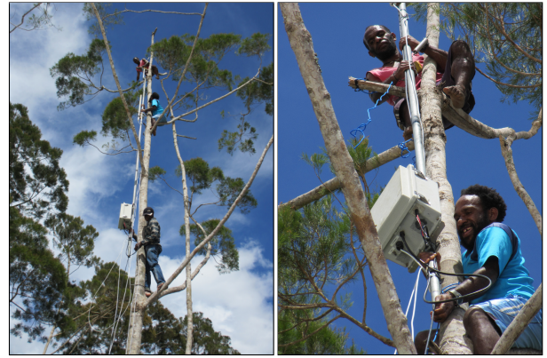
Figure 1: The CCN installation in Papua
